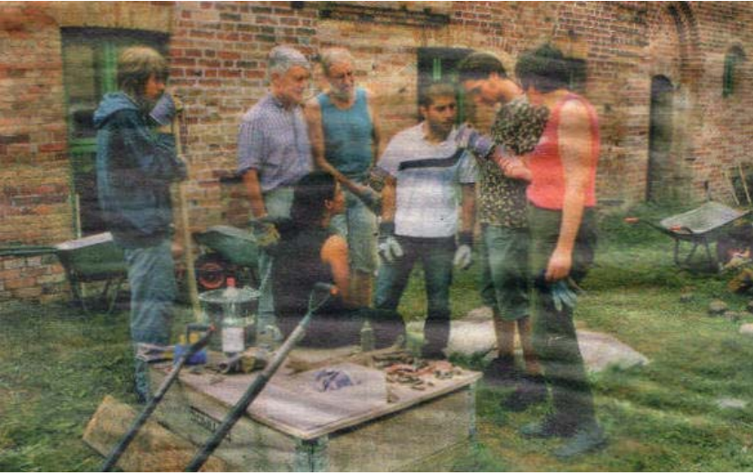
ora et labora action: preparing old walls of monastery Tempzin
